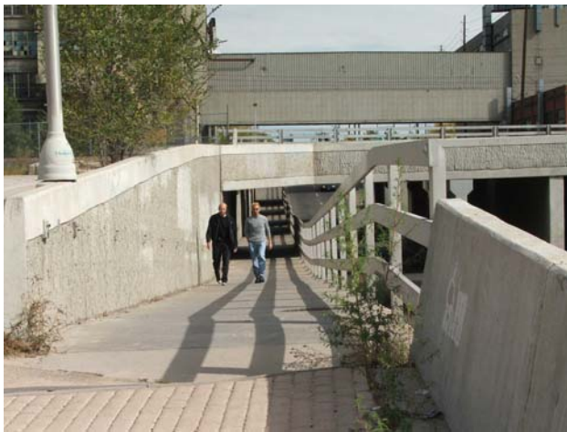
Pedestrian Underpass along Mississippi Avenue
