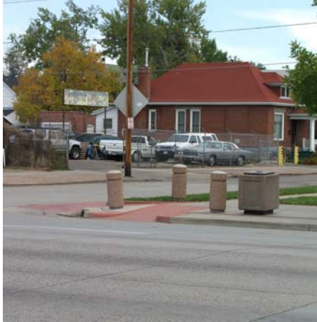
Curb Ramps along Broadway
