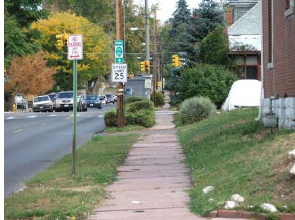
Detached Sidewalk along Exposition Avenue
