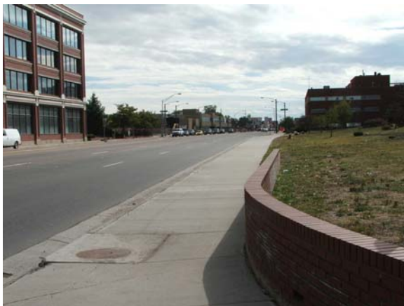
Attached Sidewalk along Broadway
