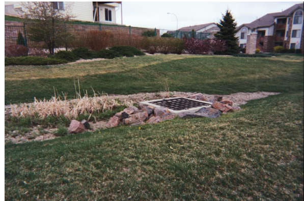
EXHIBIT 1.8 SAFE, ATTRACTIVE, MAINTAINABLE INFILTRATION BASIN
