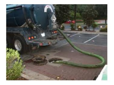
It is important that you do not treat your sinks and drains like a garbage can. Garbage disposals can overload a grease interceptor with solids, making it much less efficient and requiring it to be pumped out more frequently. Additionally, if interceptors are not pumped and cleaned out regularly, acids will form, as the grease turns septic. These acids are very destructive and over time can dissolve baffles, piping, and tank walls<sup>ii</sup>.
