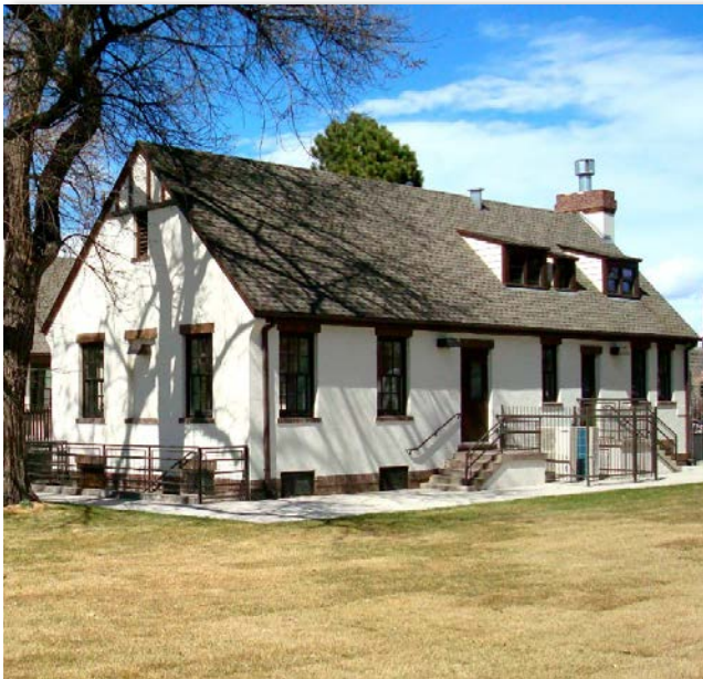
Restored exterior facade
