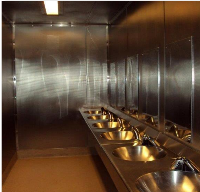
New sink fixtures and backsplash
