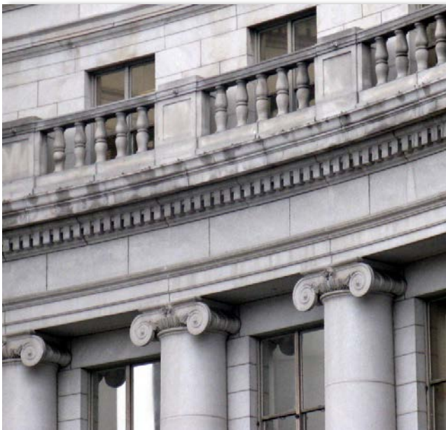
Restored masonry facade
