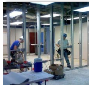
Interior wall reconfiguration
