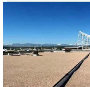
Reconstructed built-up roof
