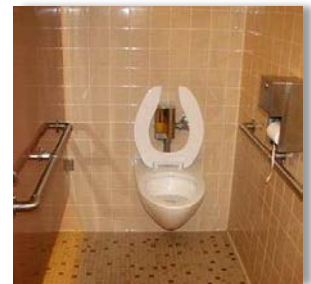
Restroom fixture improvements
