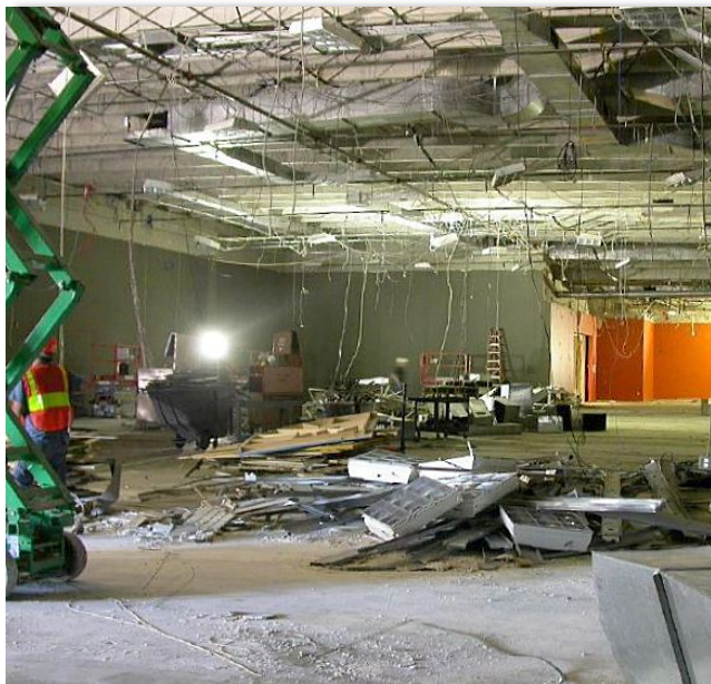
Phipps Gallery renovation
