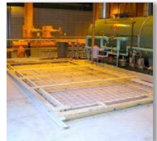
Boiler maintenance pad installation
