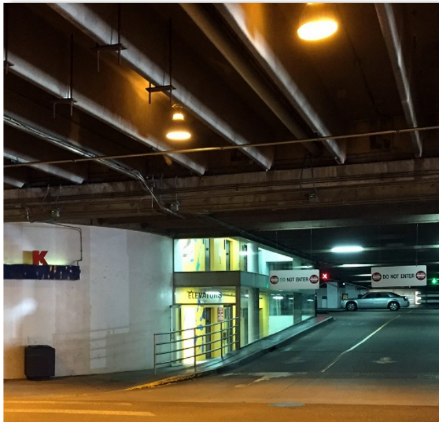
Completed structural improvements
