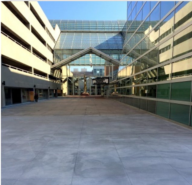
New Galleria concrete
