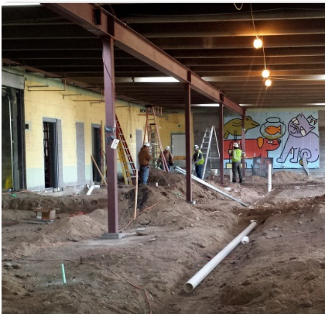
Former animal shelter decommissioning
