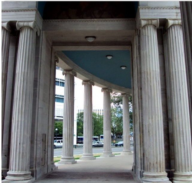
Restored Voorhies Memorial finishes
