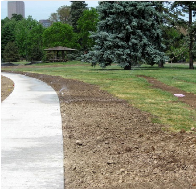
Improved irrigation system
