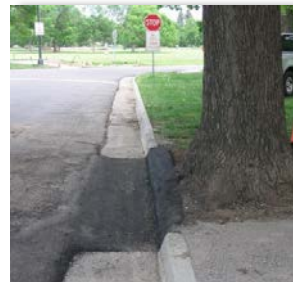
Temporary asphalt patch
