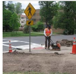
Temporary asphalt patch
