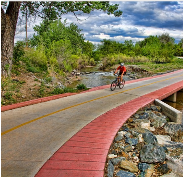
New concrete trail
