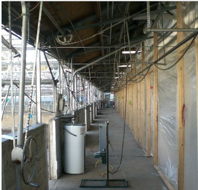
New greenhouse framing
