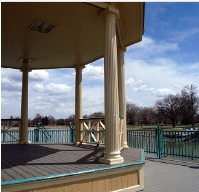
New floor deck
