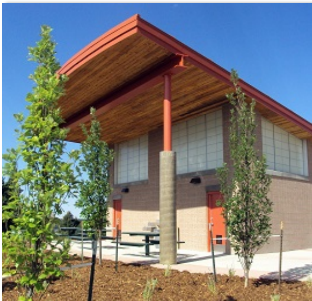
New Ruby Hill Park pavilion restroom
