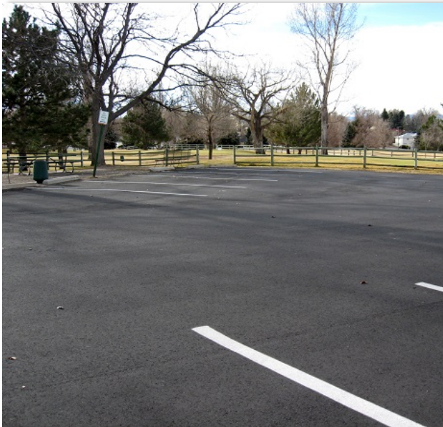
Harvard Gulch West Park parking lot improvements
