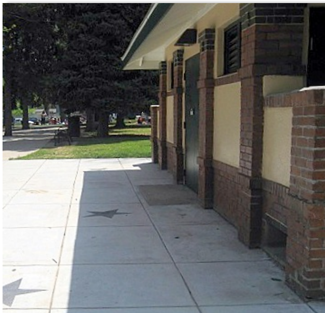
Observatory Park restroom facade
