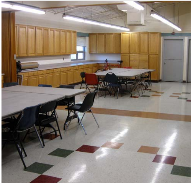
New VCT flooring
