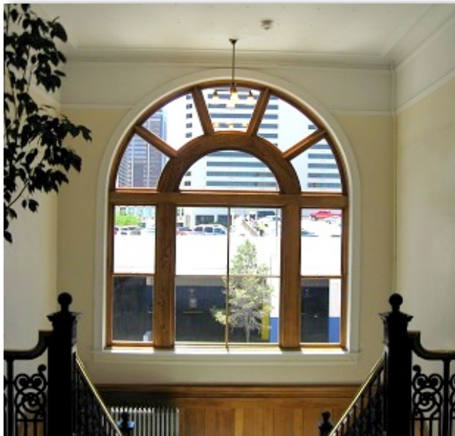
Restored interior trim
