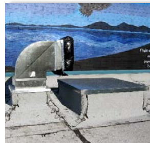
Prepared equipment base
