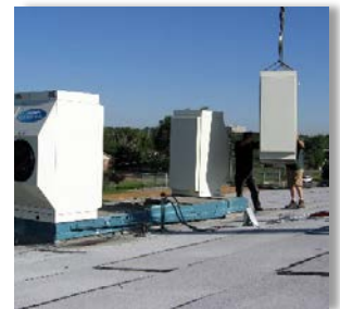
Installation of new HVAC equipment
