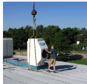
Prepared equipment base
