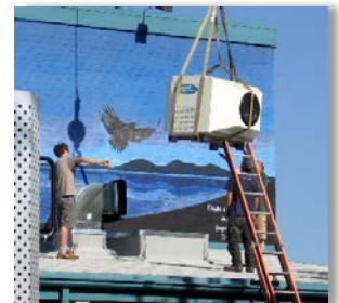
Installation of new HVAC equipment
