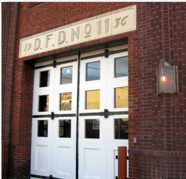
Restored fire engine doors
