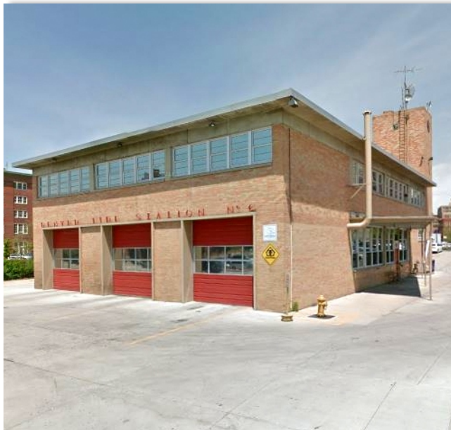
Reconstructed concrete flatwork
