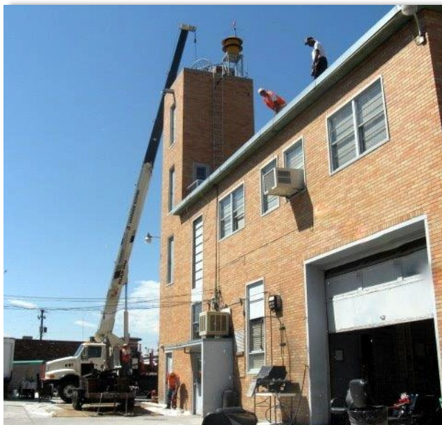
Hose tower refurbishment
