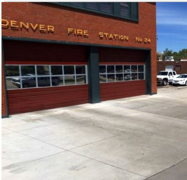
Reconstructed concrete flatwork
