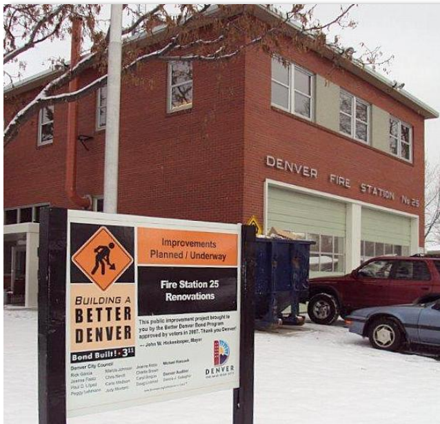
Renovation work in progress
