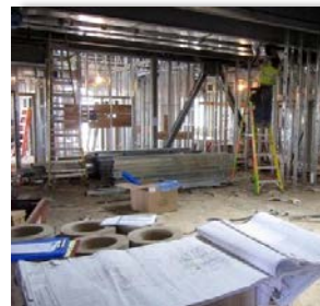
Interior wall framing
