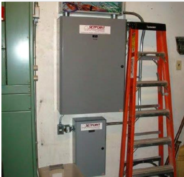
Upgrades to HVAC controls
