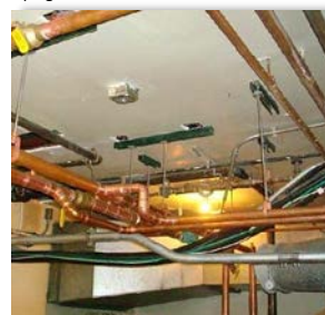
Piping installation for new boiler
