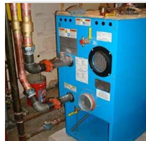
Piping installation for new boiler
