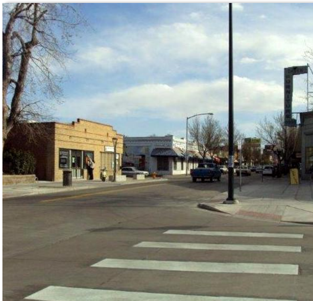
New road surface and striping
