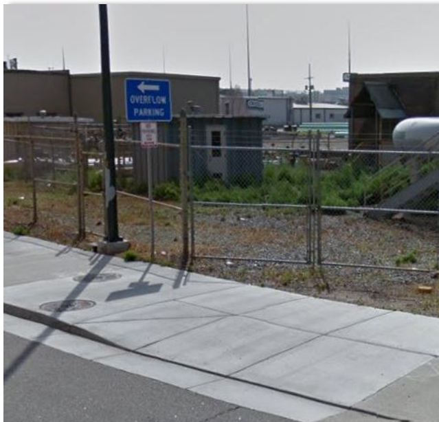
New concrete sidewalk
