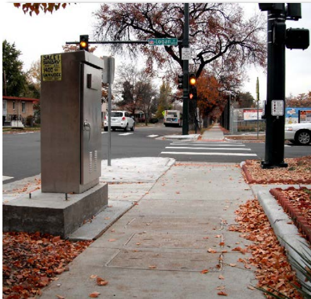
Improved sidewalks and curb ramps
