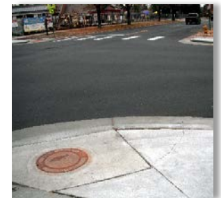
Curb extension and new crosswalk striping
