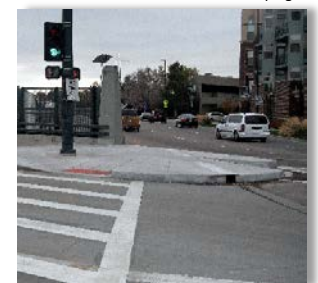
Curb extension and new crosswalk striping
