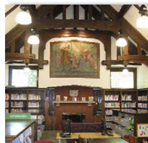
Restored wooden roof trusses
