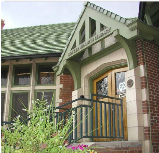
Restored exterior facade
