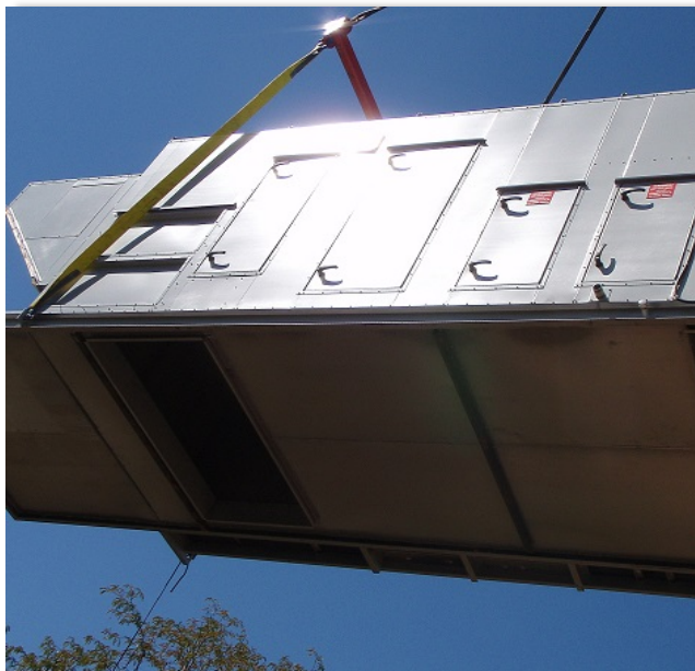
Installation of new RTU
