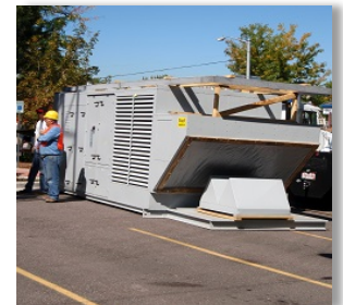
Preparation of new RTU
