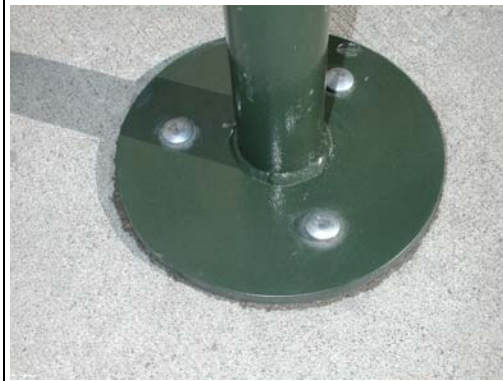
Detail of baseplate - note the vandal resistant fasteners used to anchor the rack
