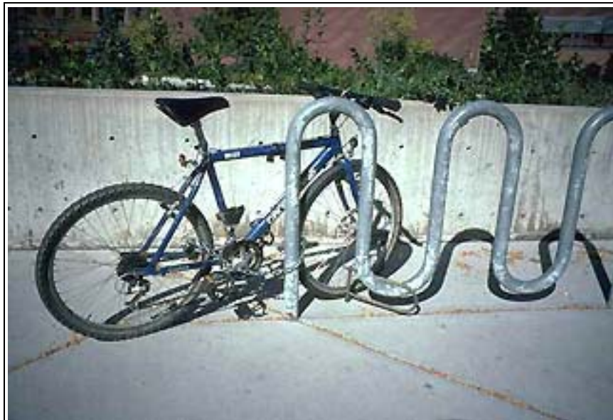
Wave type bike racks are not accepted in the City of Denver. These racks do not support the bicycle frame at two locations and are commonly used "broadside."
