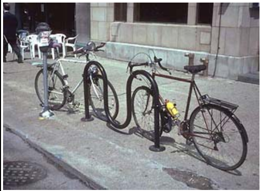
Wave type racks are commonly used "broadside" because they offer so little stability to a parked bike. The City of Denver specifies inverted U type bike racks.
