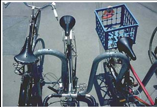
Wave type bike racks commonly have the uprights spaced too closely to provide the capacity stated by the manufacturer. Denver specifications require that inverted U type racks be used no closer than 30" on center.
