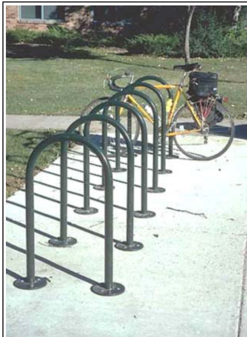
The Denver standard inverted U type bike rack supports the bike frame at two locations and allows users to secure their bikes with either a cable or U type lock.
