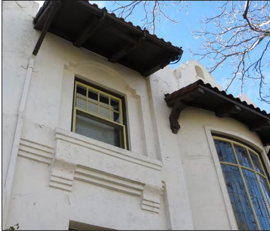
Figure 7: North (side) elevation, close-up of overhang eaves, pent roof, and bow window, photo by Mason Seymore 2016
