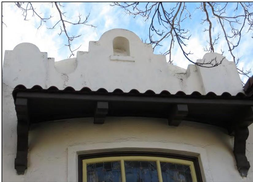
Figure 8: North (side) elevation, close-up of parapet and pent roof, photo by Mason Seymore 2016
