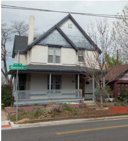
83. Use a roof form that is consistent with typical roof forms of existing structures in the district in terms of pitch, orientation, and complexity. The new house illustrated on the right uses a roof form that is typical of existing structures in the district, such as the house illustrated on the left.
