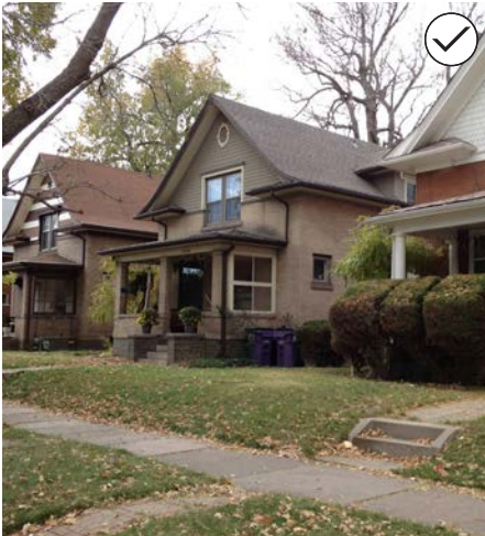
85. Locate a new building to fit within the established setback (front and side) and yard patterns seen in the historic district.
