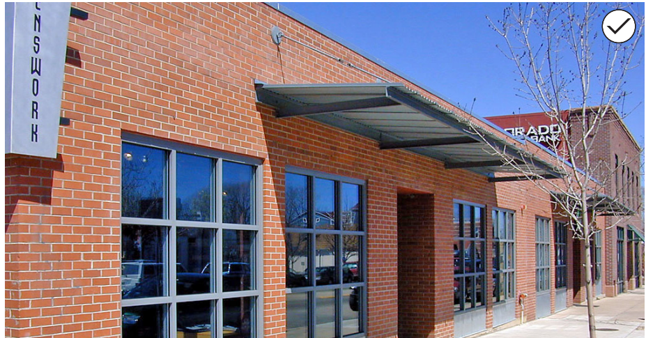
109. When introducing a new building into a historic district, it is also appropriate to consider incorporating sustainable design features that are typical of buildings in the surrounding historic context, such as canopies to provide shade.
