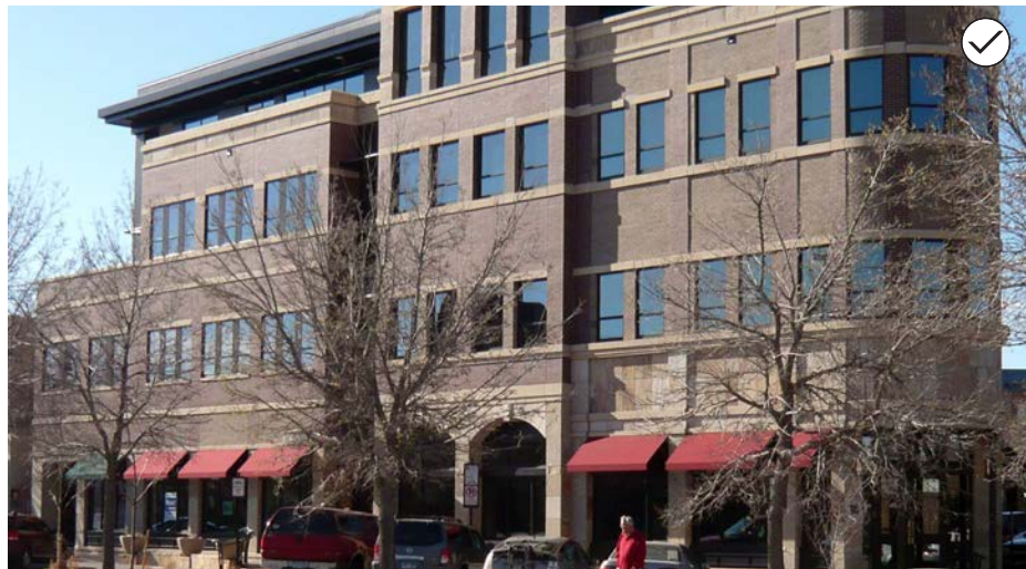
98. Use vertical and horizontal articulation design techniques to reduce the apparent scale of a larger building mass.
