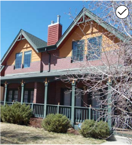
94. Use porch posts and columns that are proportioned similarly to those seen in the surrounding historic context.
