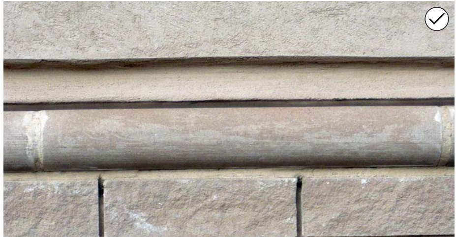
82. New materials that convey characteristics similar to historic materials may be considered if they have a similar appearance, size and shape to traditional materials, such as the cast stone illustrated above, which is detailed to convey a sense of authenticity.
