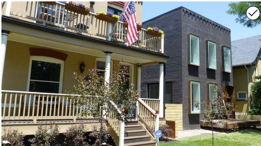
78. Design the façade to reflect typical historic proportions of height to width in the surrounding context/block.
