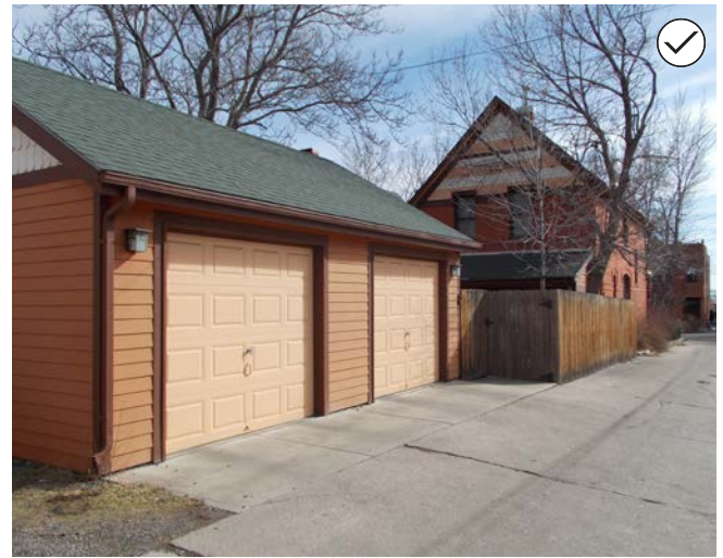
96. Design a new garage or secondary structure to be compatible with, and subordinate to, the primary structure and surrounding historic context.
