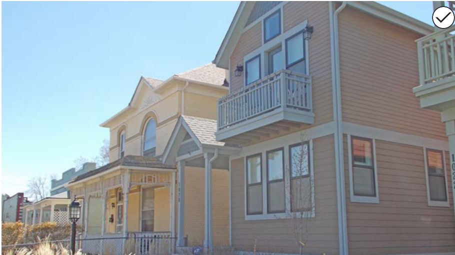
91. Use façade articulation techniques to help a new duplex, town house, or other small-scale residential building fit within the scale of the surrounding historic context.
