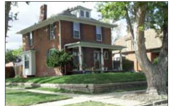
. . . and a Denver Square on Bryant.
