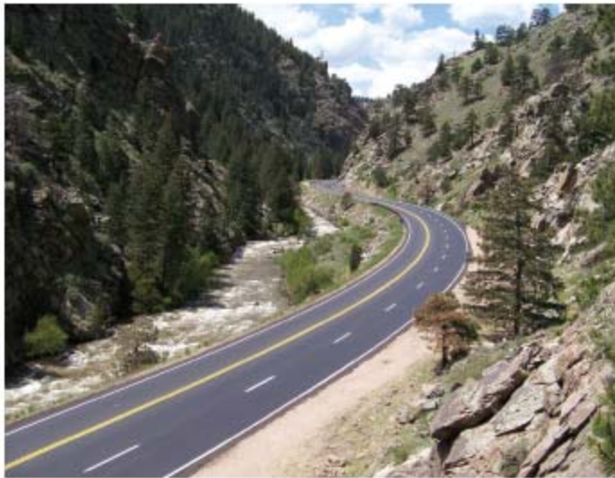
US 6 Clear Creek Canyon: rock fall mitigation
