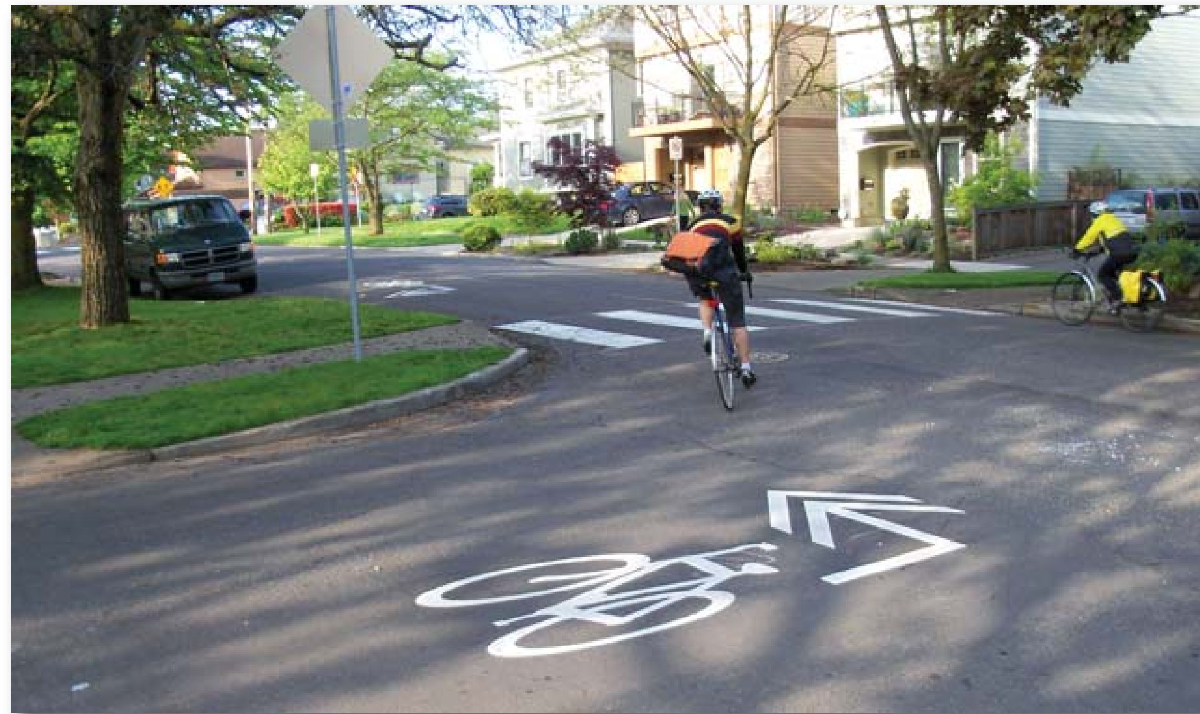
directional pavement markings guide cyclists along a neighborhood bikeway
