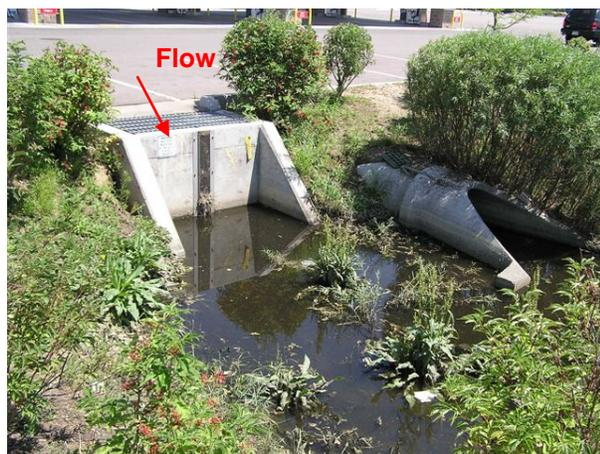
*Photo 10. Flow from this parking lot bypasses water quality treatment. The inflow pipe is also too close to the outflow. Lack of micro-pool also caused outlet clogging and standing shallow water.*
