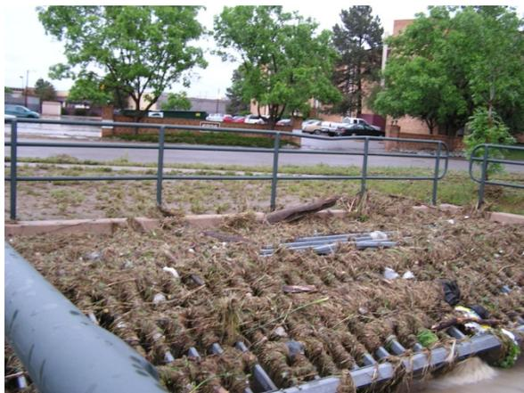
*Photo 6. Debris blocking trash rack at culvert.*
