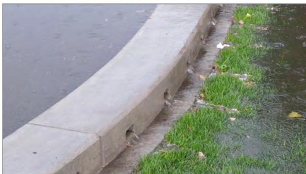
**Figure 3.4:** Example of a Denver bay at Huston Lake Denver Bays are systems that utilize standard right-of-way infrastructure (curbs, gutter, and parking areas) to create forebays that capture sediment and trash. These forebays are easily maintained by standard city practices and equipment. Stormwater then passes through small orifices in the curb into an adjacent treatment facility.
