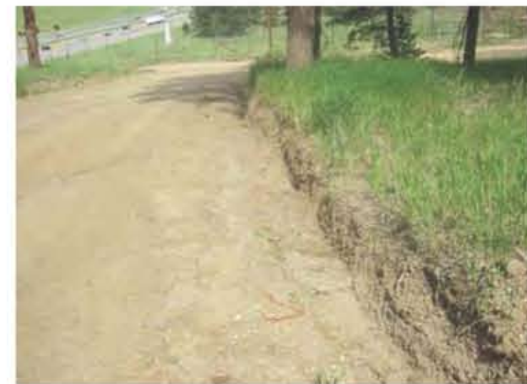
4. EXISTING ROAD CONDITIONS LOOKING EAST
