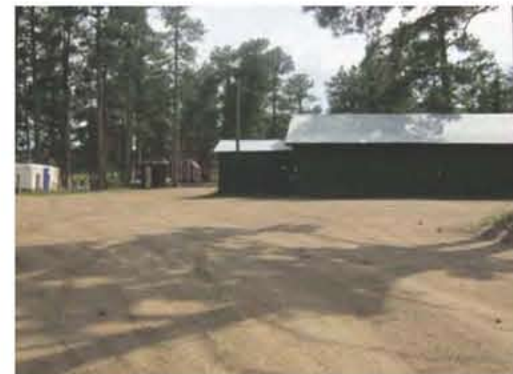
11. MAINTENANCE AREA LOOKING WEST
