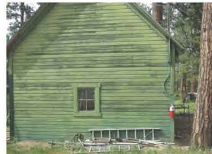
10. MAINTENANCE BUILDING BEHIND THE PATRICK HOUSE
