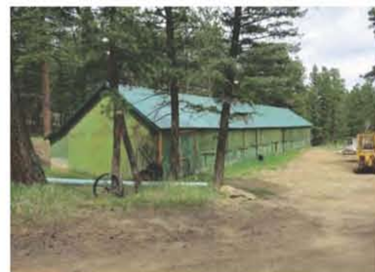
18. MAINTENANCE STORAGE BUILDING
