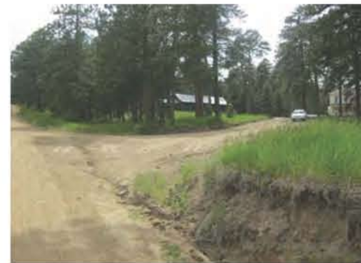
5. EXISTING ROAD CONDITIONS LOOKING SOUTHWEST
