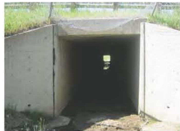
1. BISON UNDERPASS LOOKING SOUTH
