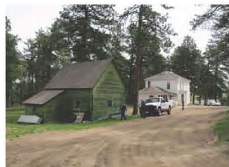
19. STORAGE SHED BEHIND THE PATRICK HOUSE
