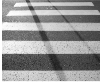
Install New Crosswalk
