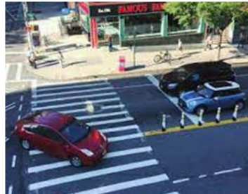
Centerline Hardening
