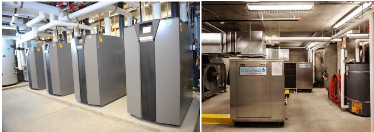
Figure 22. Central Gas Water Heating System (left) and Central Heat Pump Water Heating System (right)
