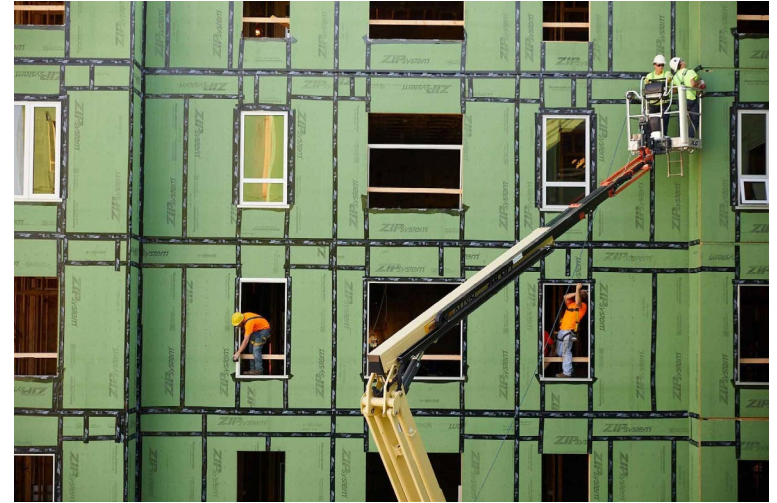
Sealing at seams and connections
