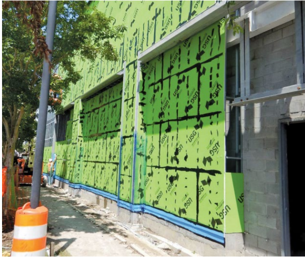
Sealing between dissimilar materials
