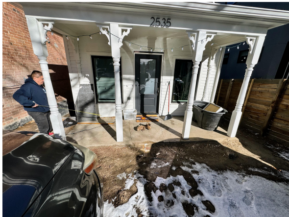
NEW FRONT OF HOUSE WITH PROPOSED WINDOWS. RECENT LANDSCAPING BLOCKS VIEW OF BOTTOM OF WINDOWS.
