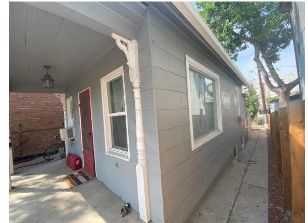
EXISTING FRONT OF HOUSE WITH EXISTING NON-HISTORIC ALUMINUM WINDOWS (RIGHT)
