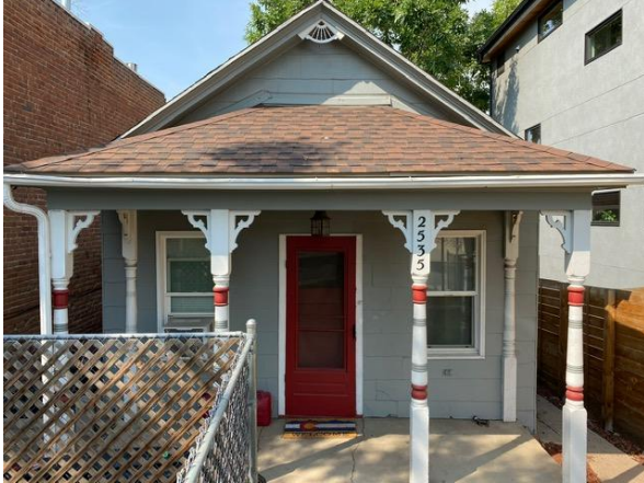
EXISTING FRONT OF HOUSE WITH EXISTING NON-HISTORIC ALUMINUM WINDOWS (CENTER)
