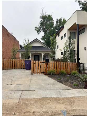
NEW FRONT OF HOUSE WITH PROPOSED WINDOW. MOST OF WINDOW BLOCKED BY LANDSCAPING.
