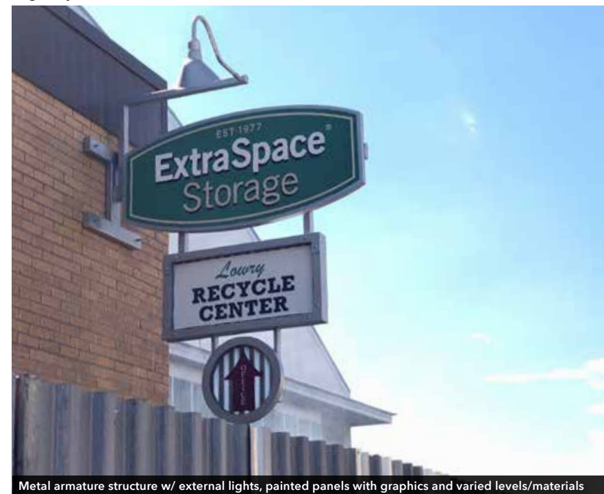
Metal armature structure w/ external lights, painted panels with graphics and varied levels/materials
