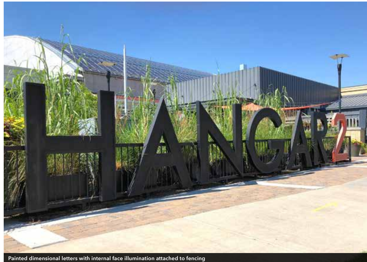
Painted dimensional letters with internal face illumination attached to fencing
