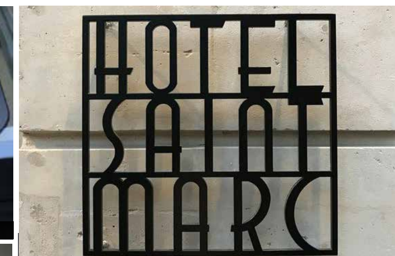
Painted flat cut letters within framing mounted with standoffs
