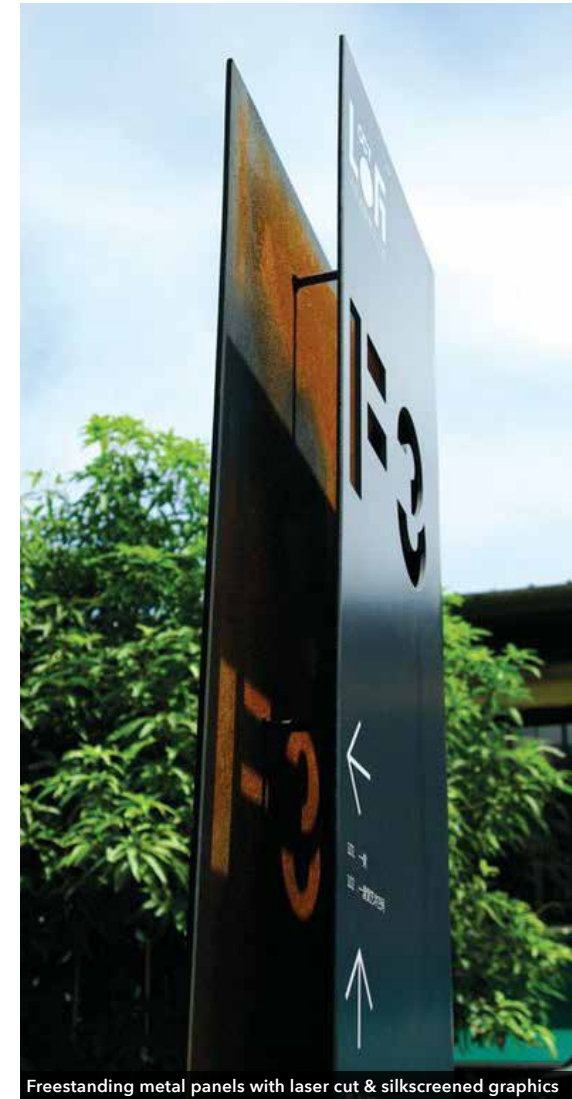
Freestanding metal panels with laser cut & silkscreened graphics
