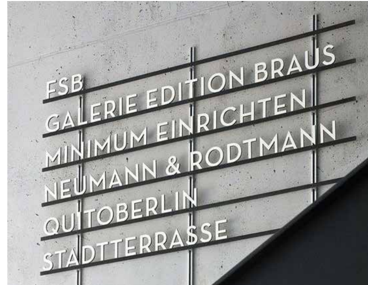
Integrated bars & letters for ease of changeability with fixed horizontal supports
