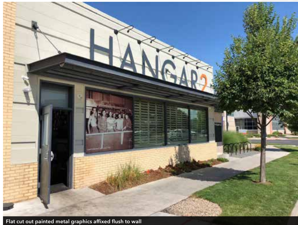
Flat cut out painted metal graphics affixed flush to wall
