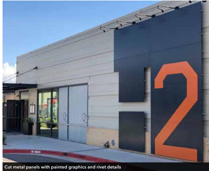
Cut metal panels with painted graphics and rivet details
