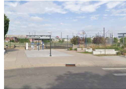
The 10th and Osage Station provide connections and access for people walking and biking
